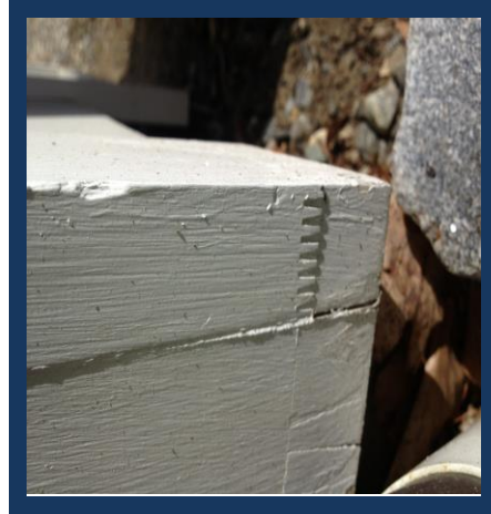
In this photo, a finger joint, this is where smaller boards have been joined together resulting in a joint that will fail in time
